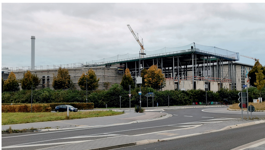
The construction of the PIC 4.0 proceeds and throws its shadow on the Campus Melaten. © IKV
